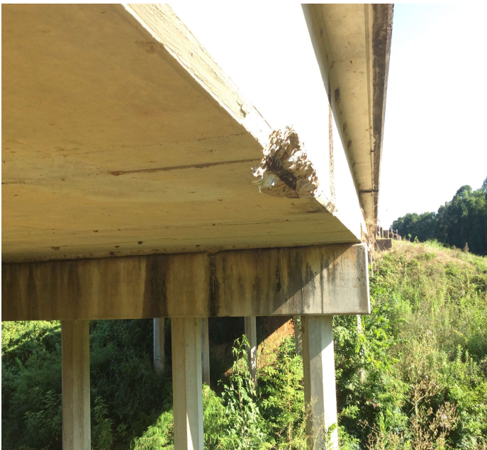
PHOTO 1 Description Rebar exposed span 3 left side edge of slab
