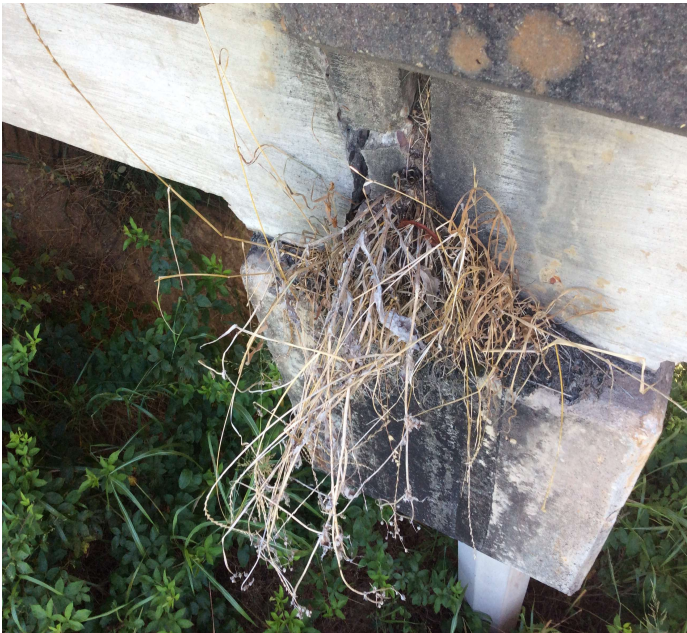
PHOTO 1 Description Bent 2 right side of slab crack
