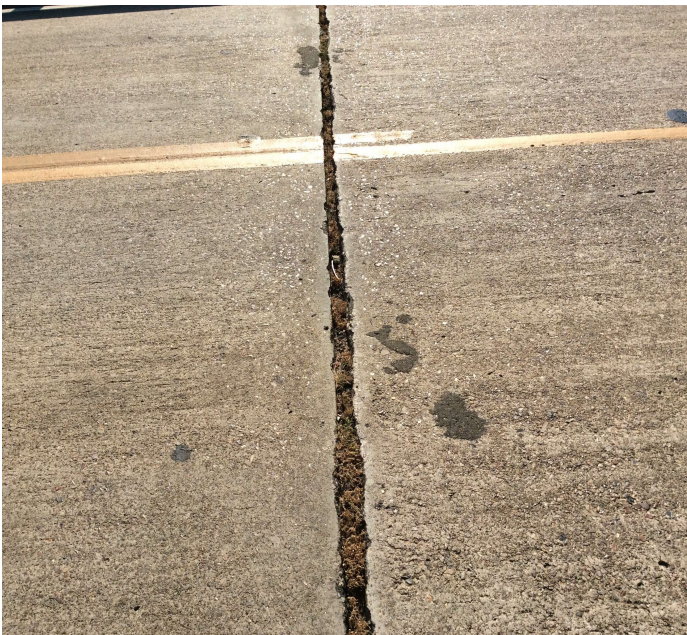
PHOTO 1 Description Joints need cleaned and refilled
