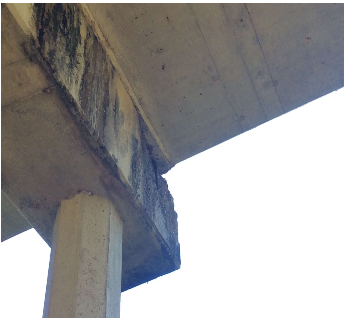
PHOTO 1 Description Spall right end of bent 3 cap with rebar exposed
